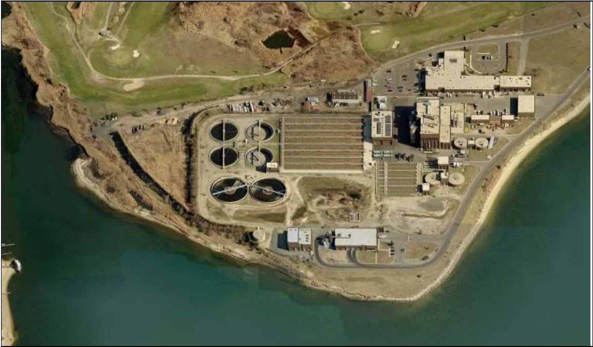
Figure 2.2 Bergen Point WWTP, West Babylon, NY
